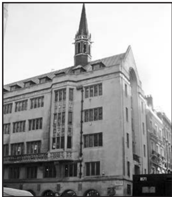
Old Bond Street Building
