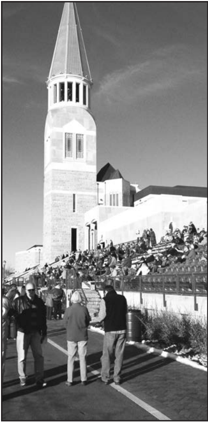
Tower and bleachers
