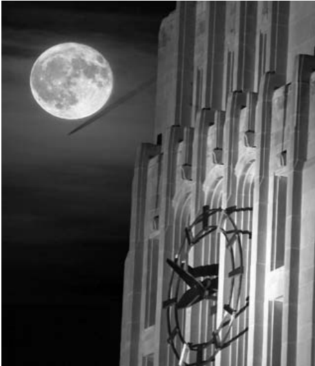
Burton Tower, University of Michigan
